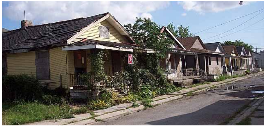
Broken homes: damaged, boarded-up houses are a stark reminder of hurricane Katrina.
